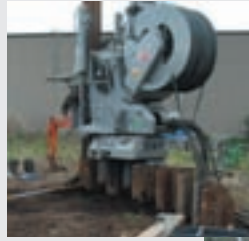
② Circular steel sheet piling
