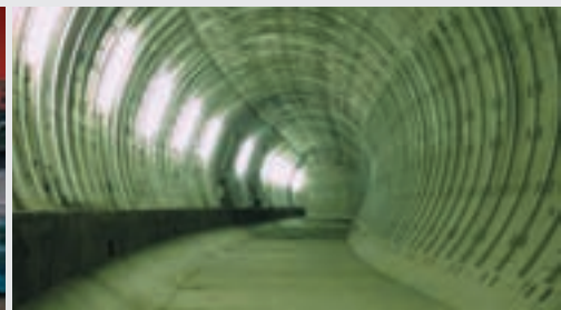
⑥ View of tunnel
