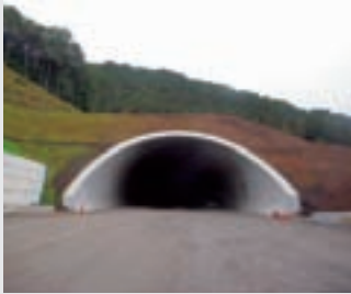
④ The Second Tomei Expressway Kanaya Tunnel
