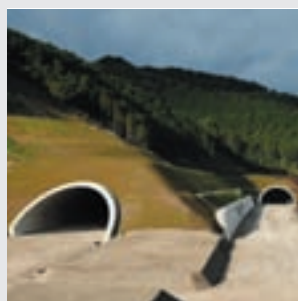
The Second Tomei Expressway: Kanaya Tunnel East Construction Work
