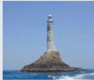
⑤ Mizunoko Shima Lighthouse (Oita Prefecture)
