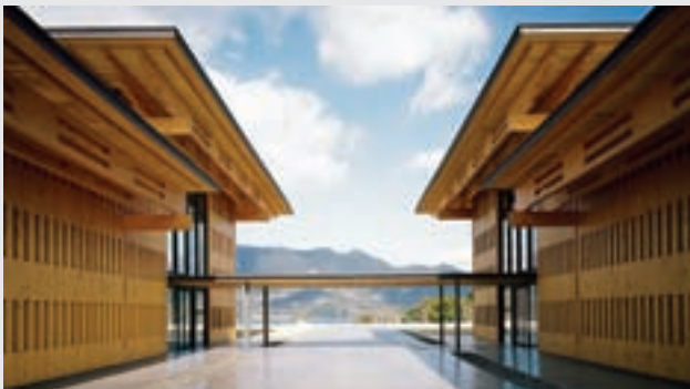
⑥ Exterior of the Kumano Kodo Center (corridor section)
