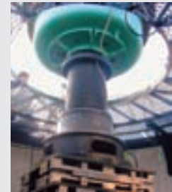
⑤ Seismic isolation device for Class 3 lighthouse lens
