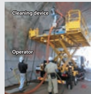
Status of demonstration tests
