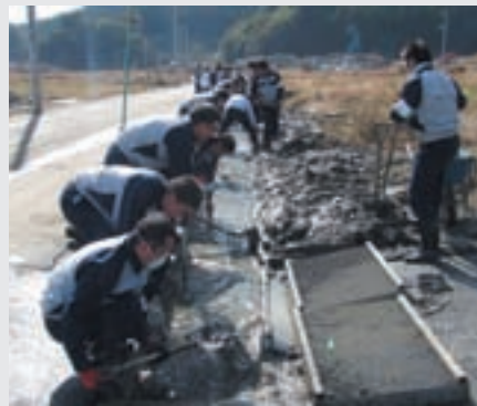
⑤ Cleaning up the gutters
