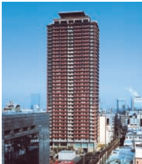
Plané Renai Springs Tower Osaka
