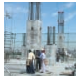
Installation of eco columns
