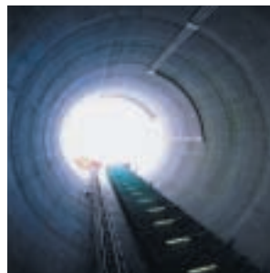
Tunnel construction for the contour drainage canal at the Oh-otoshi-Furutone River
