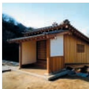
Restoration work for the Ohashi Roka of historic Wakayama Castle
