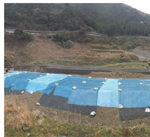
写真-7 CSG材の貯蔵
