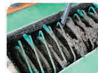
[Photo] Pouring: The concrete is poured in the spaces in between.
