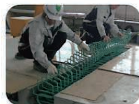
[Photo] Spiral rib insertion: The spiral rib is inserted between the loop ribs from the top.
