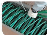
[Photo] Fastening: The spiral ribs and loop ribs are securely fastened.
