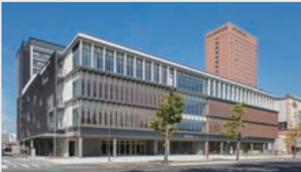
Wakayama-Jo Hall Work period: July 2019 to December 2021 Structure: SRC (partially steel and RC) Total floor space: 14,279.86 m 2
