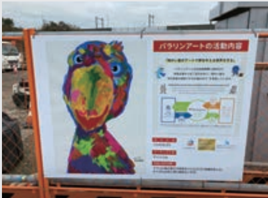
Railway construction site (Miyagi Prefecture)
