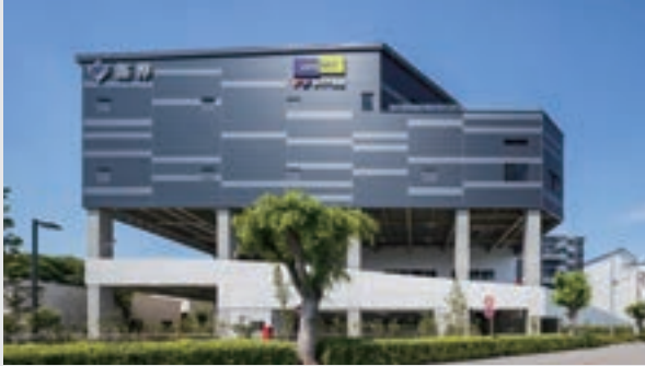
Landport Koshigaya Work period: February 2019 to May 2021 Structure: RC and steel Total floor space: 31,980.95 m 2
