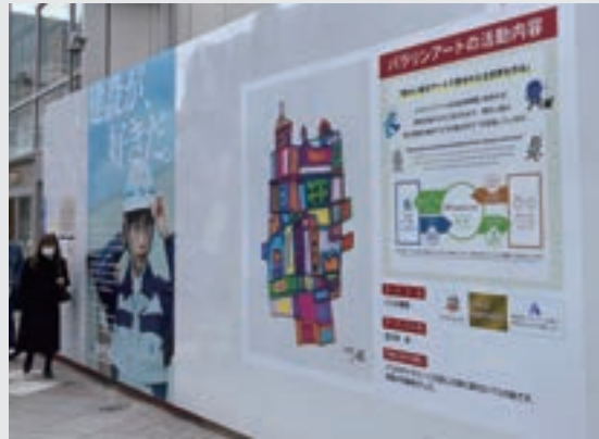
Condominium construction site (Tokyo)
