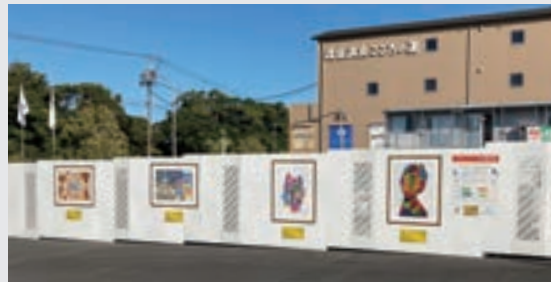
Construction site of a local government building (Kagoshima Prefecture)
