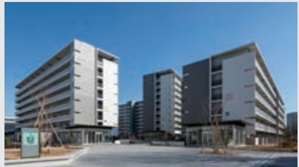
Toyoshikidai Apartment Complex Work period: February 2020 to February 2022 Structure: RC Stories above ground: 8 Total units: 142
