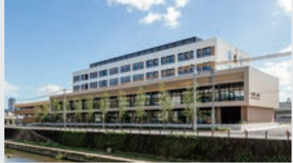
Manazuru-kai Medical Corporation's Kokura Daiichi Hospital Work period: May 2020 to September 2021 Structure: steel Total floor space: 13,697.86 m 2
