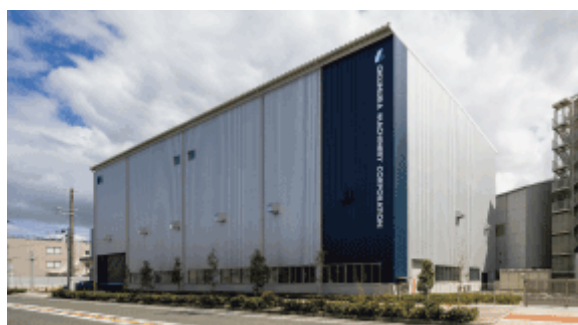
Exterior view of Okumura Machinery Corporation's No. 4 Plant (Osaka-shi, Osaka)
