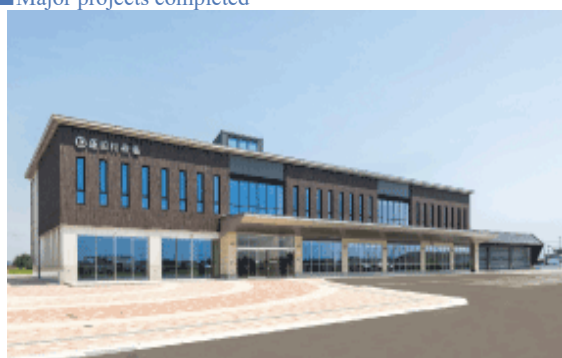
Yomogita Village Office (Higashi Tsugaru District, Aomori Prefecture)
