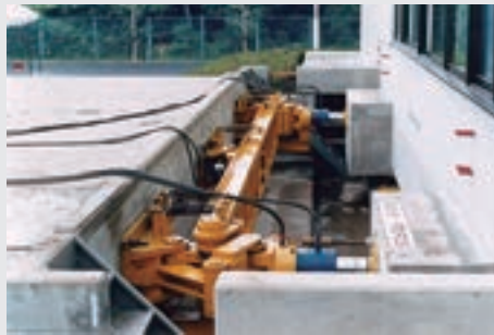
② Installing jacks to force horizontal movement of the building
