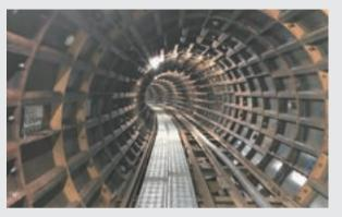
Construction of Futtsu-Chiba High-voltage Main Line Work period: July 2018 to May 2022 Kisarazu shield tunnel: 2,212 m, Obitsugawa shield tunnel: 2,398 m, Anesaki shield tunnel: 1,390 m, Kaneda shield tunnel: 2,555 m
