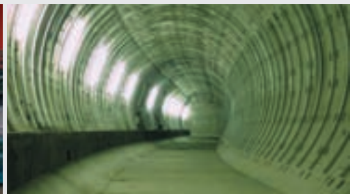
⑥ View of tunnel
