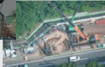
② Construction site (aerial view)
